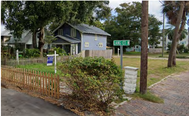
South end of Lang's Bungalow Court
