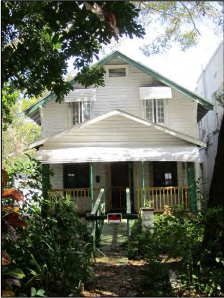
Figure 7: 345 Lang Ct N, 2 story front gable. Visual mass is mitigated by smaller front porch
