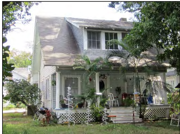
Figure 6: 349 Lang Ct N, 1.5 story side gable
