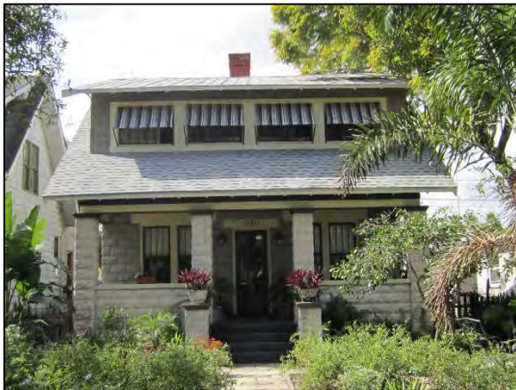
Figure 5: 336 Lang Ct N, 1.5 story side gable
